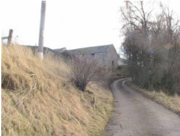
Fig. 2 : Existing watermill structure, as viewed from the approach.
