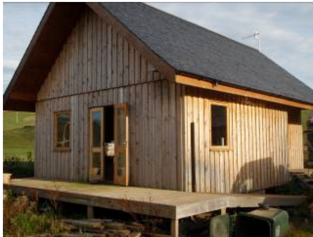
Fig. 3 : Existing 'cabin' accommodation
